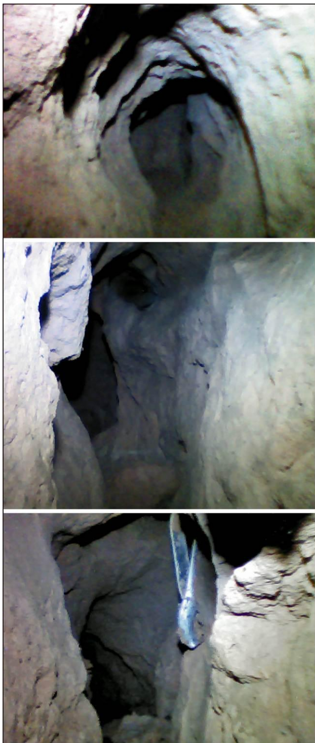
Fig. 9: Pictures of the tunnels linking the craters of the Strauch property. Picture at the bottom shows the auger inside one of the tunnels and illustrates the difficulty to hit the narrow tunnels at 3 meters depth.
