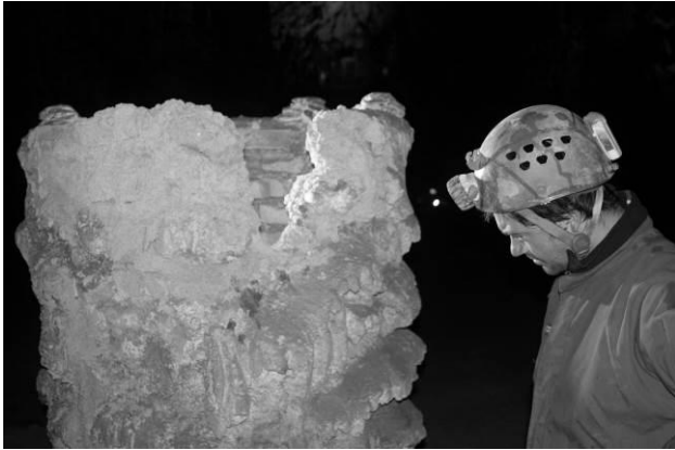
Fig. 3: Hidden electric installations, Postojnska jama cave. Photo by: Rosana Cerkvenik
