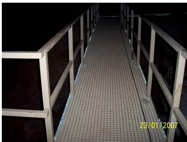
Fig. 20 – The emergency lights placed along the edge of the pathway in the Grutas de Bustamante, Mexico
